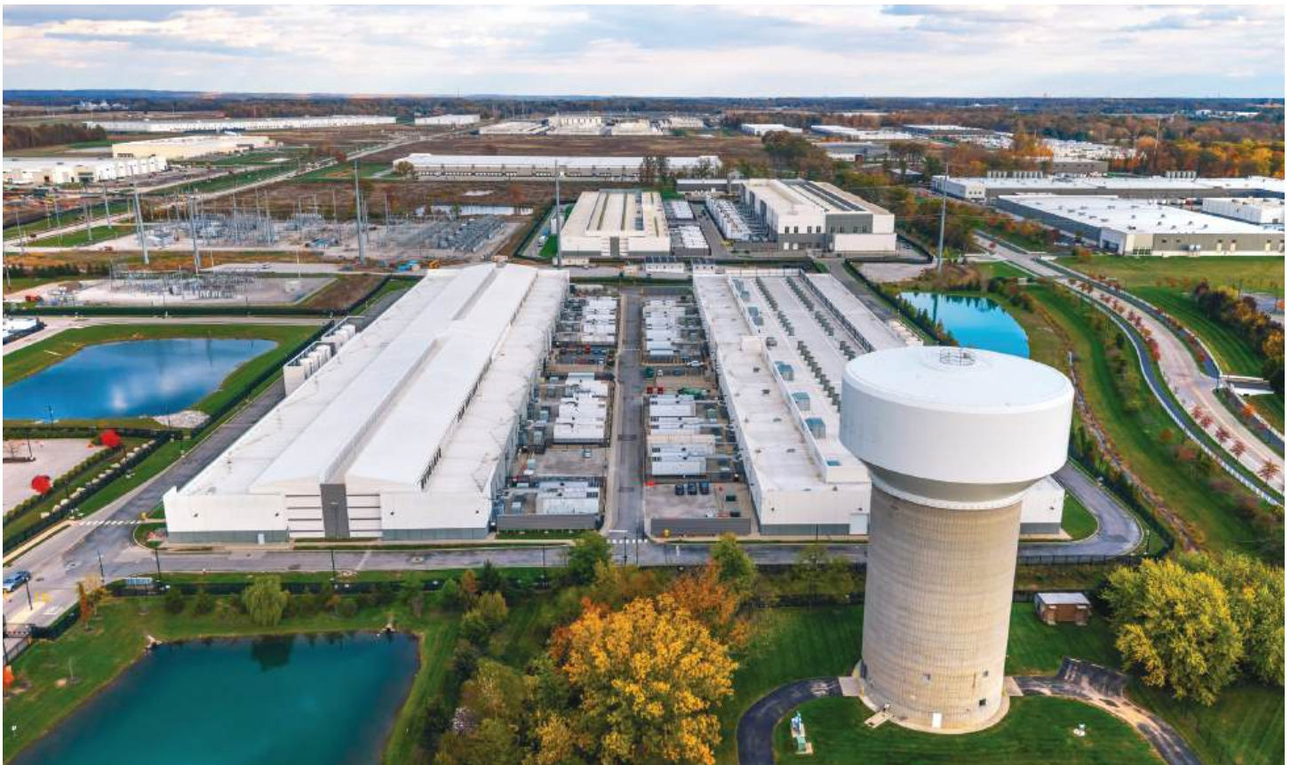
Figure 1. AI and cloud infrastructure data center facility.
