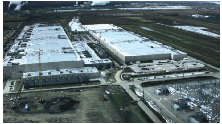
Figure 5. Google Data Center, Council Bluffs, Iowa
