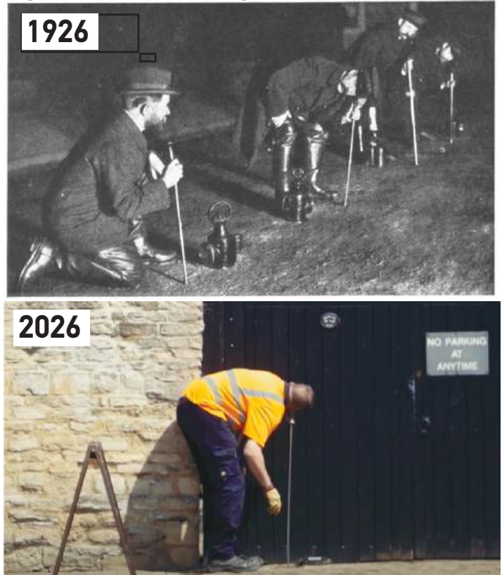
Figure 11. The role of listening sticks to find leaks, continues.
