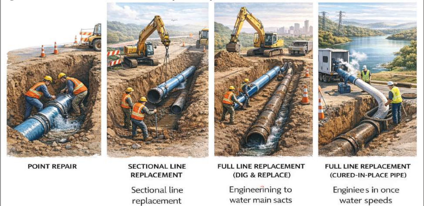
Figure 39. Common Methods for Water Main Repairs & Replacement
