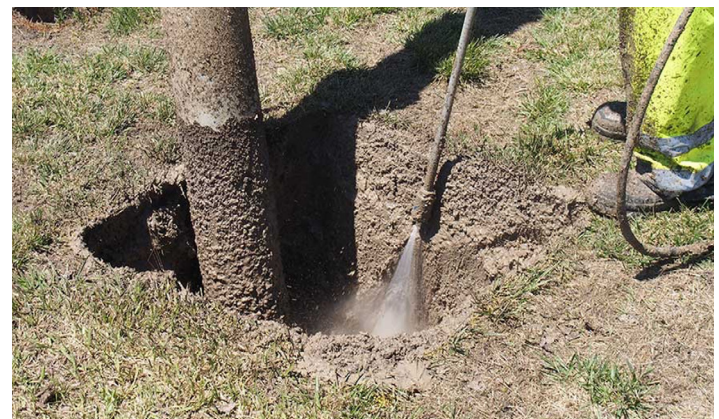
Figure 8. Removing topsoil using hydro-excavation.
