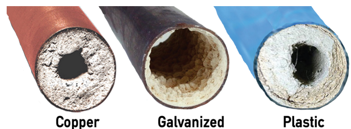
Figure 2. Scaling in Copper, Galvanized, and Plastic pipes.
