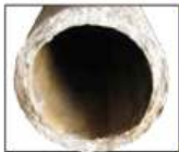
Asbestos Cement Pipe
