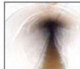
Cured-In-Place Pipe
