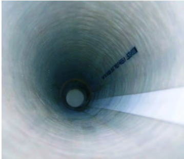
Post-CIPP, Pre-Lateral Reinstatement
