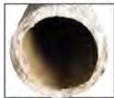
Asbestos Cement Pipe
