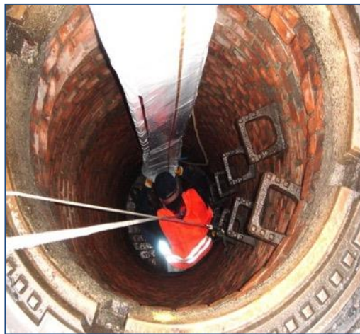
Liner winched in place (NO scaffolding need)
