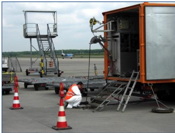
Control unit for UV-Light Curing (NO boiler requirement)
