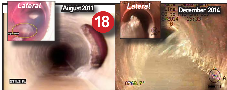
18. Mis-Reported Bad Reconnection. Same Leak, 4 Years Running.
