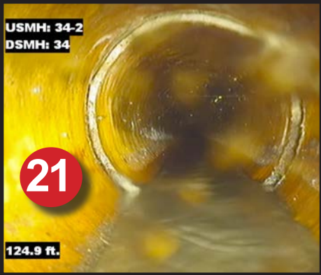
21. Post-CIPP Misaligned / Open Joint
