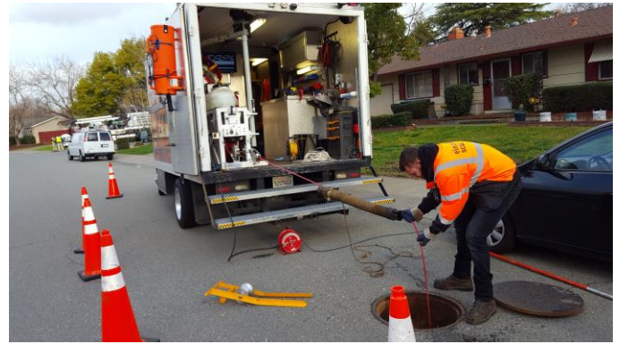
Electro Scanning Inspection locates within 1 cm and measures in water volume per second each crack, fracture, bad joint, hole, defective service connection, or any other opening. Photo by Electro Scan Inc.
