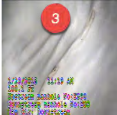
1. Post-CIPP, Bad Service Reconnection. Heavy Roots. 2. Post-CIPP, Bad Service Reconnection. Infiltration. 3. Wrinkles. They May Leak!
