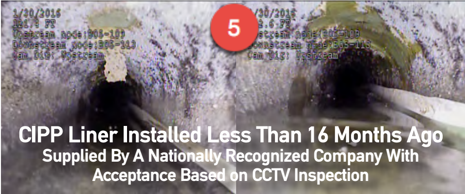
5. Bad Resin. This pipe was relined in 2014 and certified by CCTV Inspection.
