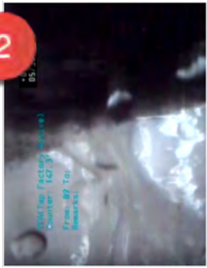
1. Post-CIPP, Bad Service Reconnection. Heavy Roots. 2. Post-CIPP, Bad Service Reconnection. Infiltration. 3. Wrinkles. They May Leak!
