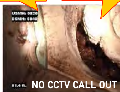
Crack in Pipe
