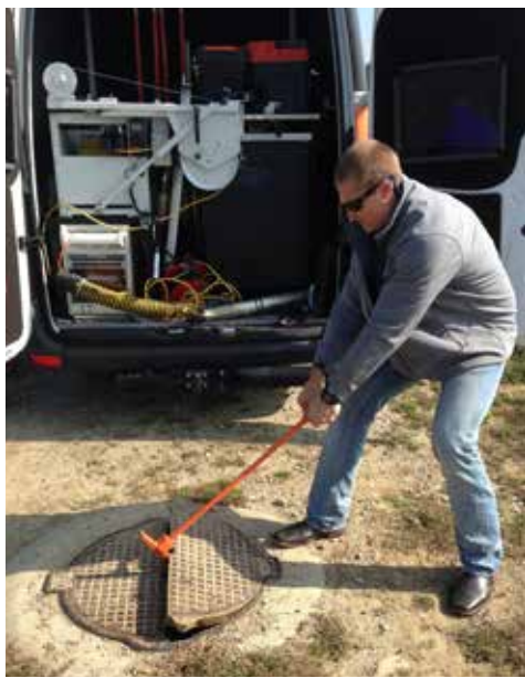
Brandon Harlow opens a Swiss manhole with his American-made 'pook'—i.e. a pick & hook.
