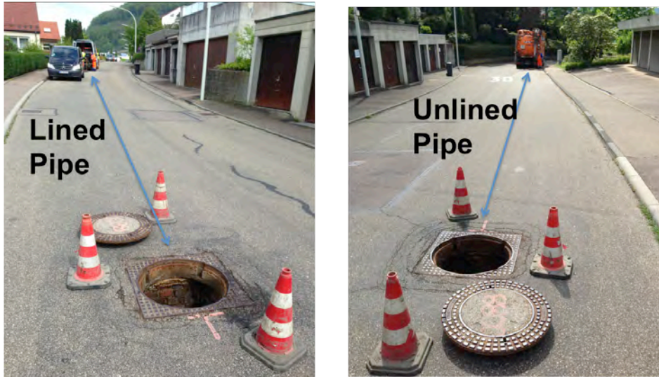
Figure 21. Field photographs of upstream and downstream segments having lined and unlined pipe, respectively.
