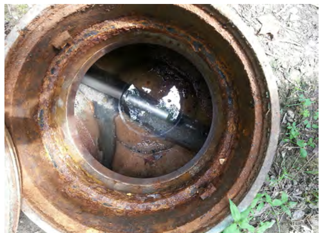
(Above) Prism Contractors & Engineers, guides water into sewer main to surround Electro Scan's moving funnel plug.
