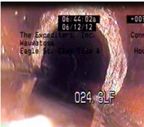
(Above). This pipe with CCTV images of three (3) joints were correctly cataloged in accordance with NASSCO's PACP standards with 'Light to Medium Encrustation'; it also passed its Hydrostatic Testing holding water pressure within standard; however, Electro Scan found all leaks. Until encrustation become an approved rehab method, these pipes need to be relined or repaired to prevent infiltration.
