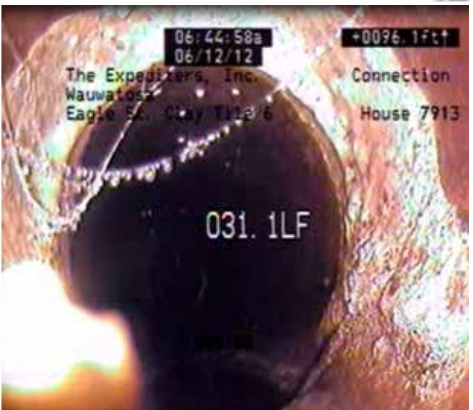
(Above). This pipe with CCTV images of three (3) joints were correctly cataloged in accordance with NASSCO's PACP standards with 'Light to Medium Encrustation'; it also passed its Hydrostatic Testing holding water pressure within standard; however, Electro Scan found all leaks. Until encrustation become an approved rehab method, these pipes need to be relined or repaired to prevent infiltration.
