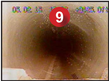
9. Missed Lateral Reinstatement
