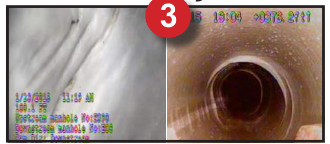
3. Wrinkles. They May Leak!
