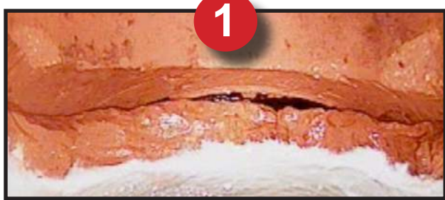
1. Post-CIPP, Bad Service Reconnection.
