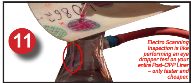
11. Defective/ Porous/ Weak Liner
