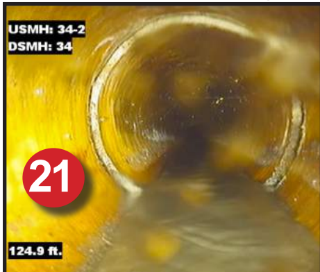
21. Post-CIPP Misaligned / Open Joint
