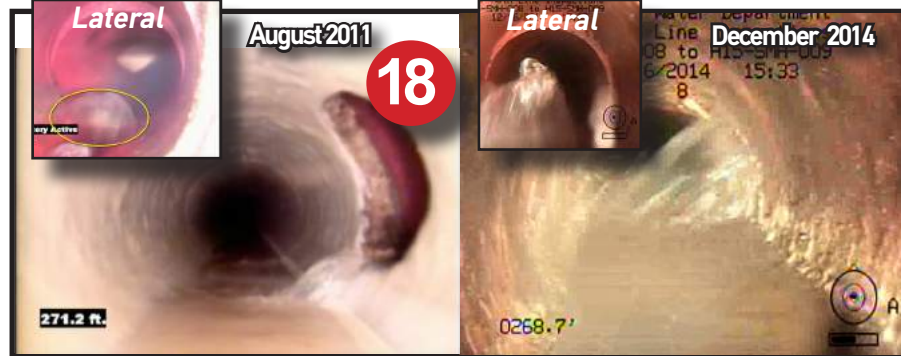
18. Mis-Reported Bad Reconnection. Same Leak, 4 years running.
