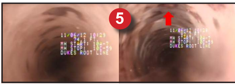
5. Infiltration Spotting and Staining
