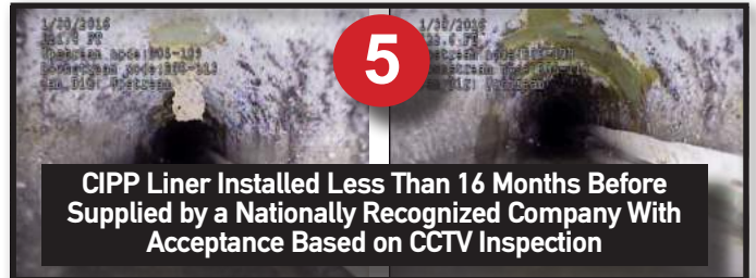
5. Bad Resin. Installed less than 16 months prior.
