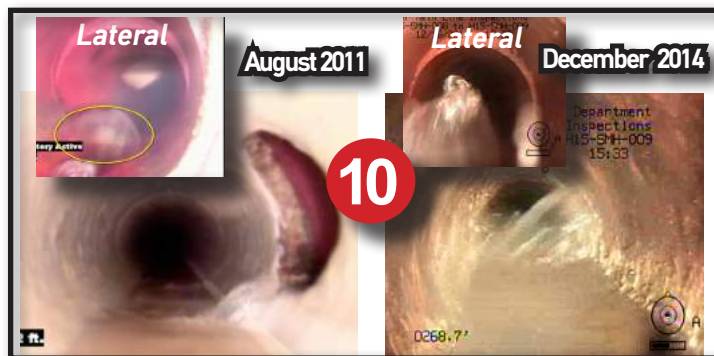
10. Misreported Bad Reconnection. Same Leak Running 4 Years.
