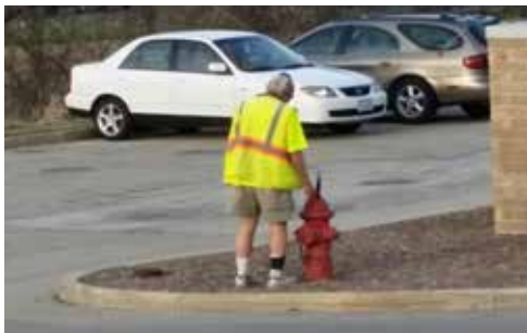
Pictured above a modern day (2015) acoustic leak detection conducted by a Great Lakes Region water utility. A contract worker attaches a hydrophone listening device for under 60 seconds to find leaks. At least it is fast, easy, and inexpensive. And, no leak was found.
