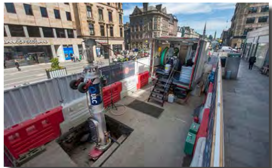
ULC's CISBOT travels under George Street, Edinburgh, Scotland repairing 1,920 feet of gas pipe.
