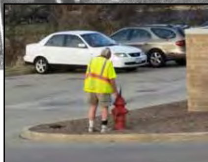
Pictured above a modern day (2015) acoustic leak detection conducted by a Great Lakes Region water utility. A contract worker attaches a hydrophone listening device for under 60-seconds to find leaks. At least it is fast, easy, and inexpensive. No leak found.
