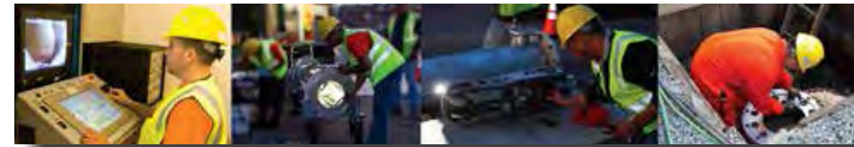
Pictured above: CISBOT, the cast iron joint sealing robot, from ULC Robotics internally sealing leaking joints inside a cast iron gas main
