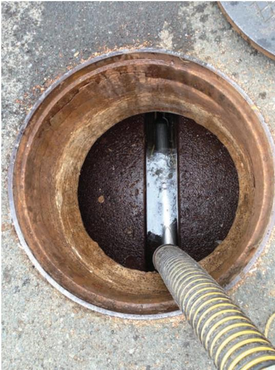
**The Electro Scan probe releases a focused array of low-voltage high-frequency electrical current, of only 10 volts and 40 milliamps, which locates and quantifies all defects in non-conductive sewer mains and laterals. Most sewer pipe materials are electrical insulators. A defect in the pipe that leaks water will also leak electrical current.**
