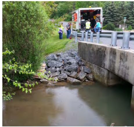
Figure 5: Scanning the PVC pipes adjacent to the creek, which was suspected to be the cause of the pipe infiltration.
