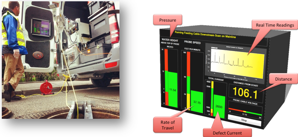
Figure 16. Data automatically displayed on Operator's Real Time Console, requiring no data entry or interpretation during scanning process.
