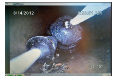
This push camera image shows the probe up at the inflatable plug. This is where the scan will start. The camera will be removed, water put in the pipe, and then the probe will be withdrawn through the water as it completes its scan.
