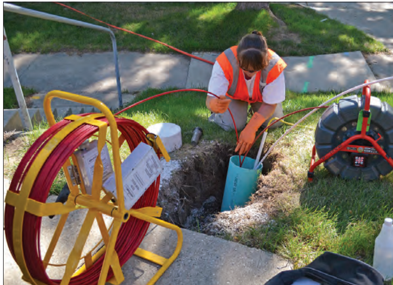
Elizabeth Gruell of Brown and Caldwell inserts the probe into the lateral via the cleanout, pushing it to the end of the section of pipe to be scanned.
