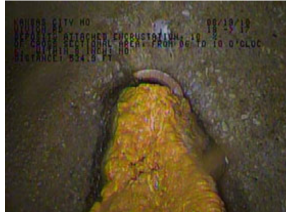
Figure 6-12. Encrustation Deposit Between SMH 18 and 17 Digital Scan (Multi-sensor) (left), CCTV(right).
