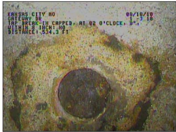
Figure 6-12. Encrustation Deposit Between SMH 18 and 17 Digital Scan (Multi-sensor) (left), CCTV(right).
