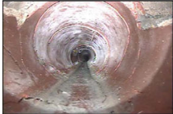
(b) Grade 2 Circumferential Fracture in MH 125-127
