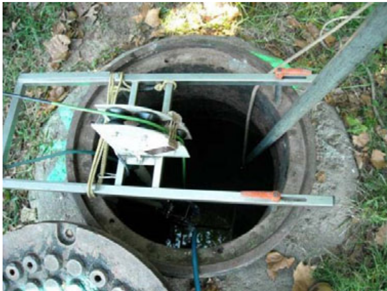
Figure 4-10. Electro-scanning Cable Guide Set-up at Manhole Opening.
