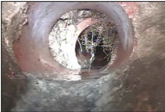
(a) Grade 2 Off-set joint in MH 136-137
