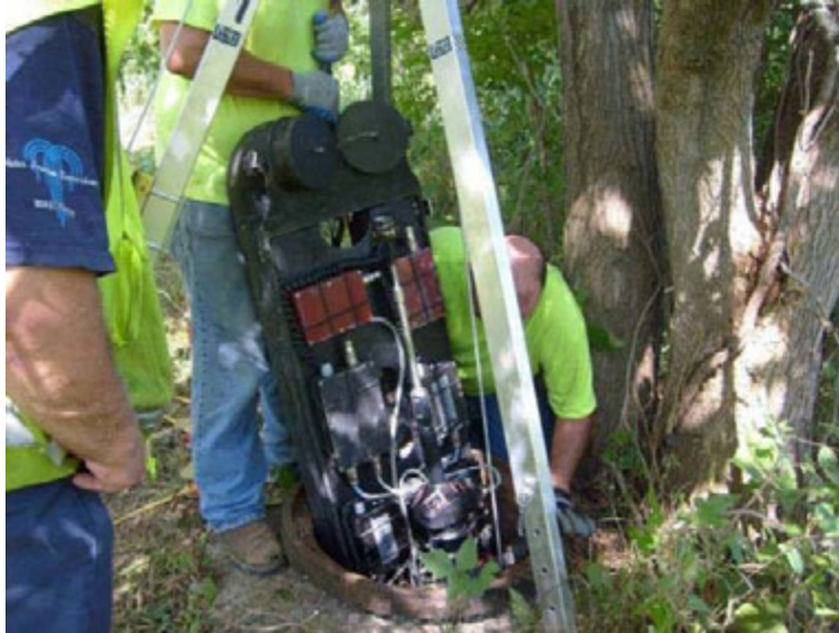
Figure 4-13. Lowering Multi-sensor Float into SMH 3 at Start of Work.
