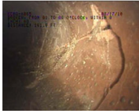
(b) Broken Pipe, Grade 5 Defect
