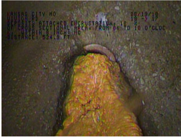
(a) Encrustation Grade 2 Defect
