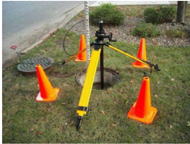
c) Lowering tripod at deep manhole.
