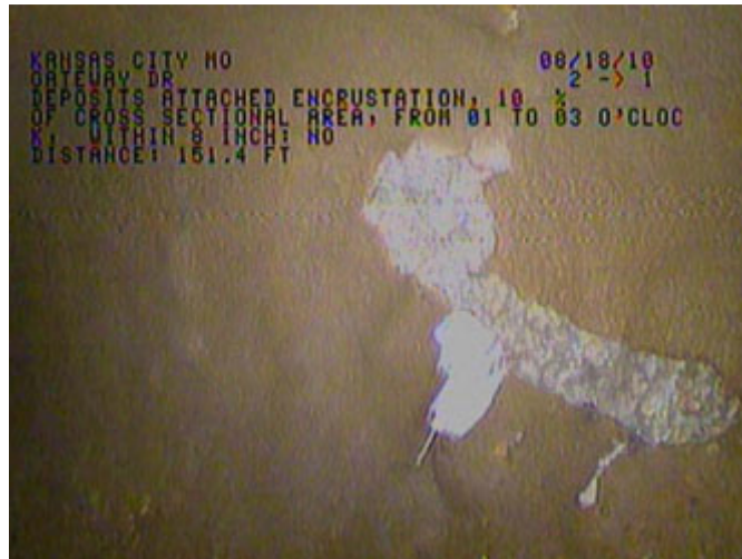
Figure 6-15. CCTV Data 150-ft Downstream of MH 2 Showing Encrustation Deposit.
