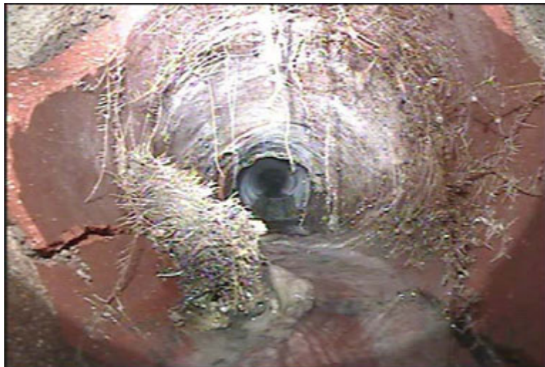
(c) Grade 3 Broken Pipe in MH 127-128
