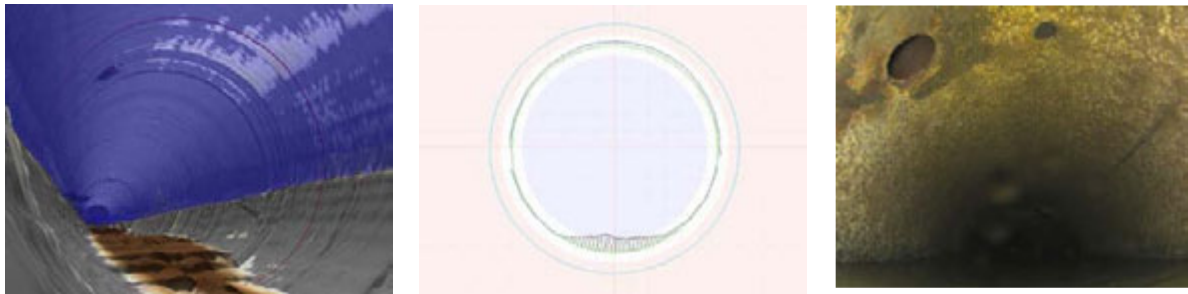
(a) 3D image at 518.1-ft (b) cross-sectional graphic at 517-ft (c) HD image of the pipe crown at 516.5-ft.
