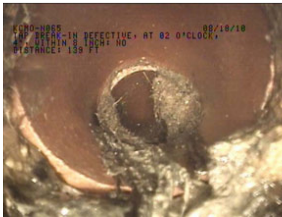
(c) Defective Tap, Grade 3 Defect
