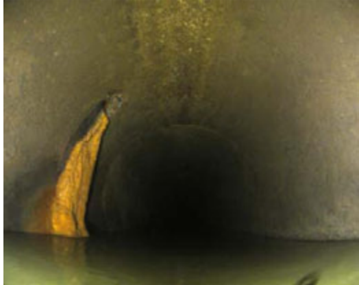
Figure 6-12. Encrustation Deposit Between SMH 18 and 17 Digital Scan (Multi-sensor) (left), CCTV(right).
