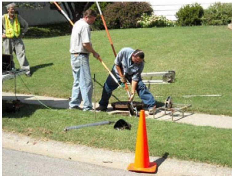
Figure 4-9. Retrieval of the Sewer Cleaning Hose During Electro-scanning Inspection.
