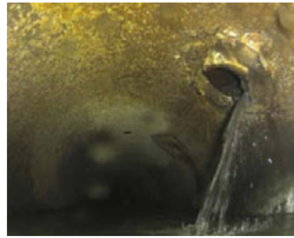
Figure 5-14. Cross-Sectional and HD Images of 2.5-in. Protruding Lateral at 528.4-ft.
